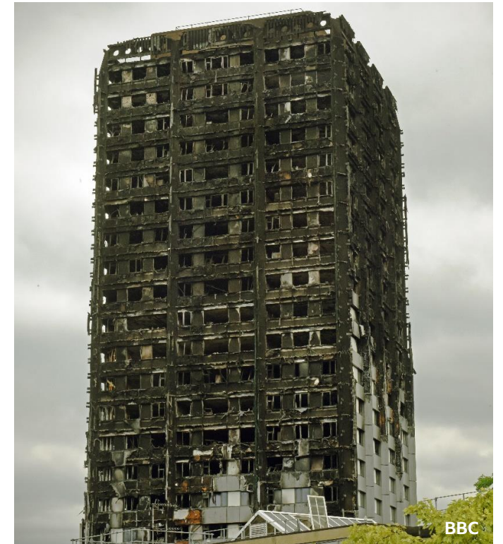
Grenfell Tower in London, two weeks after a fire engulfed the building in June 2017, killing 72 people
